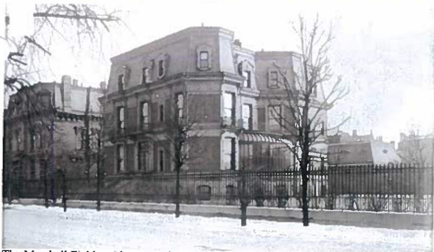
The Marshall Field residence at 1905 Prairie Avenue (demolished). DN-0003324, Chicago Daily News negatives collection, Chicago History Museum.
